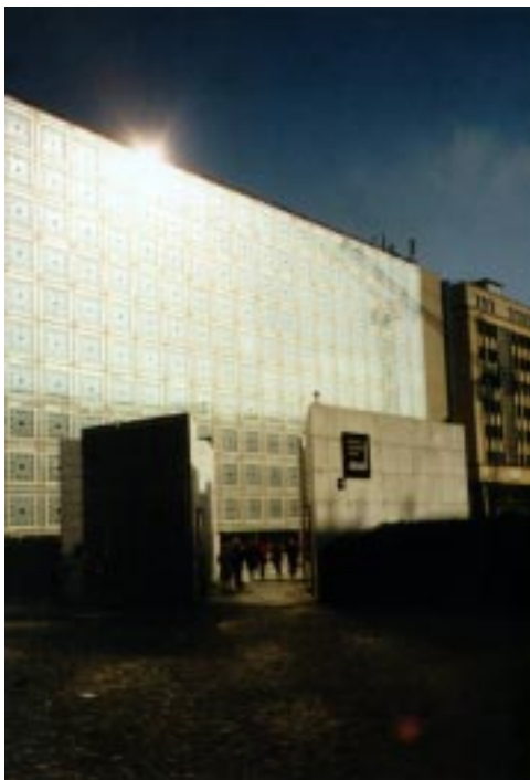
Figure 9: Arab Institute, south facade.
