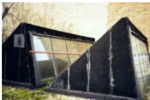
Figure 18: Maison Planeix, exterior view of
